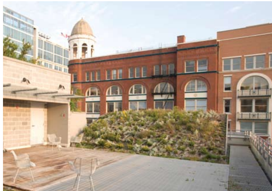
Green roof on the headquarters of the American Society of Landscape Architects in downtown D.C.
