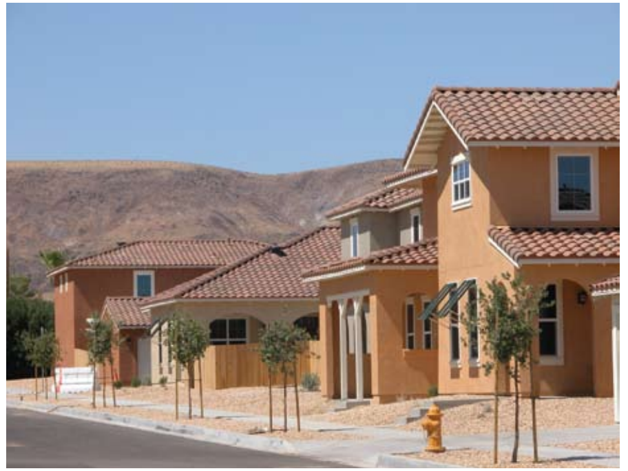
At Fort Irwin, Calif., revitalized military housing achieves a 50 percent reduction in energy usage over standard design and construction methods.
