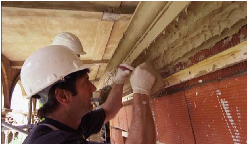
Formal building wall section built using aerated clay block.
