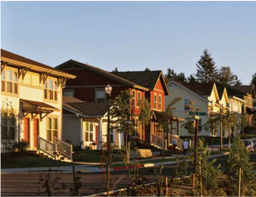
Salishan in Tacoma, Wash., where 91 percent of the runoff is treated and infiltrated through bioswales.
